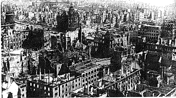
The aftermath of the Allied air raids on Dresden, February 1945.
